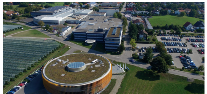
mayr ® headquarters in Mauerstetten
